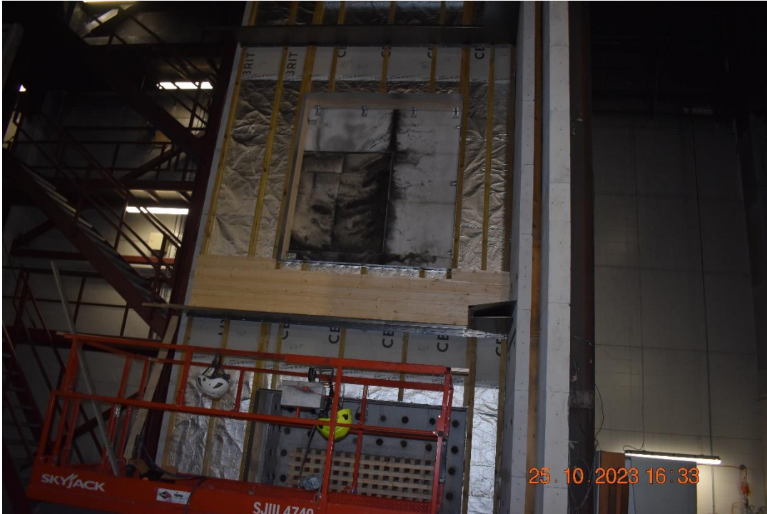
Photo No. 13 Horizontal cladding is being mounted.
