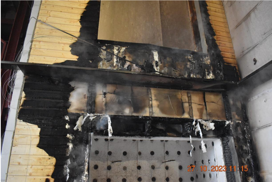
Photo No. 29 Test specimen after the test. Detailed photo of cladding between the fire chamber and the first window.
