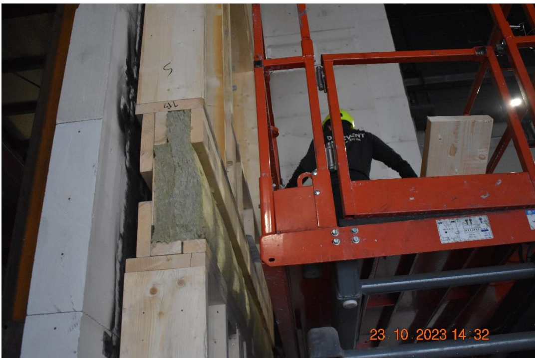
Photo No. 4 Insulation in the gap.
