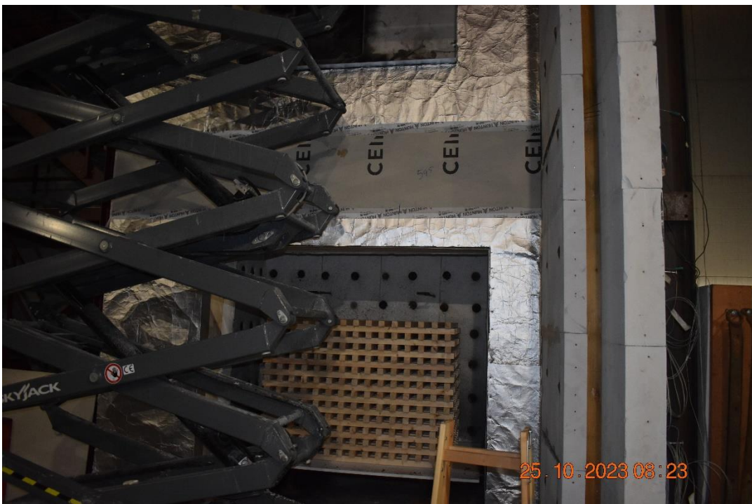
Photo No. 8 Cembrit boards mounted to the gap.
