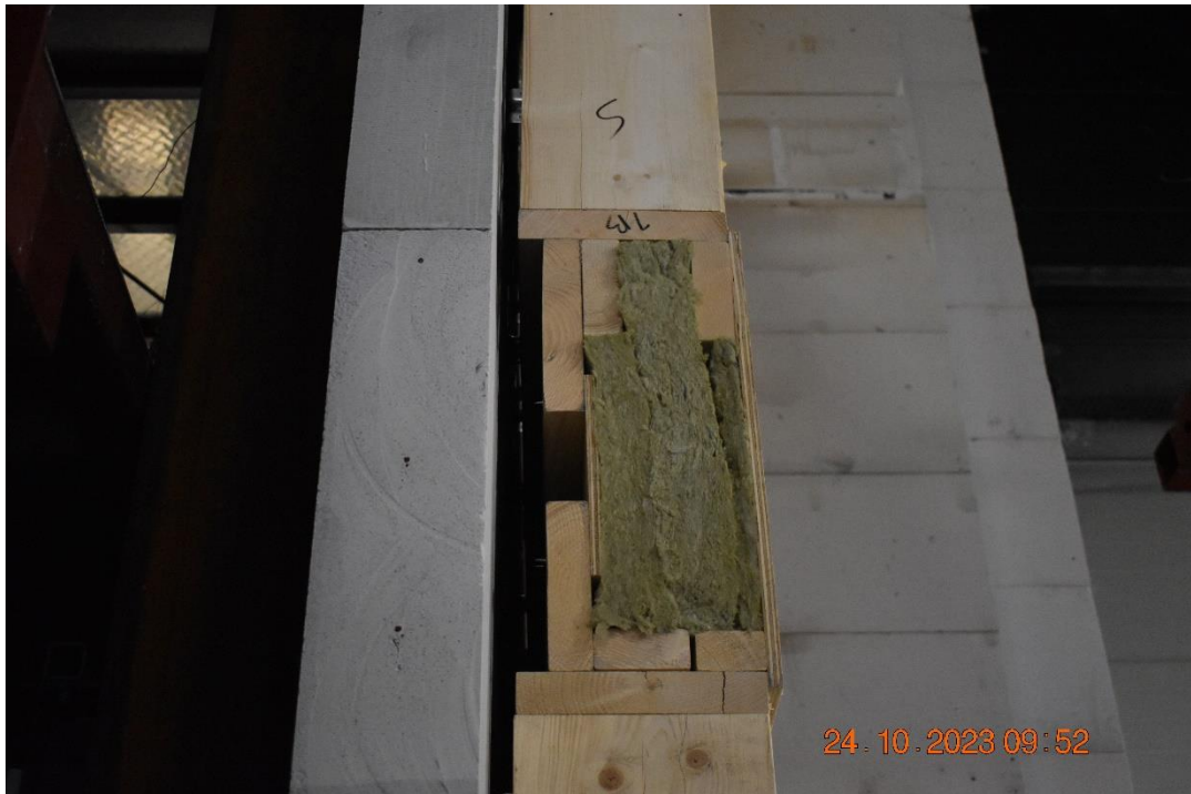
Photo No. 6 Plywood on the gap to keep the insulation.
