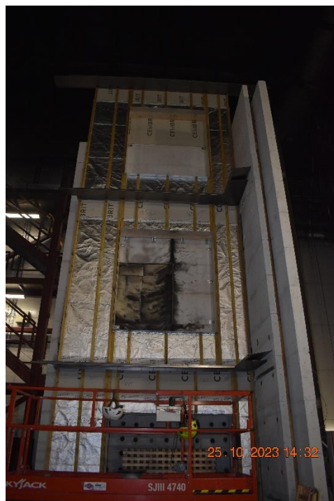
Photo No. 12 Vertical formworks have been mounted.
