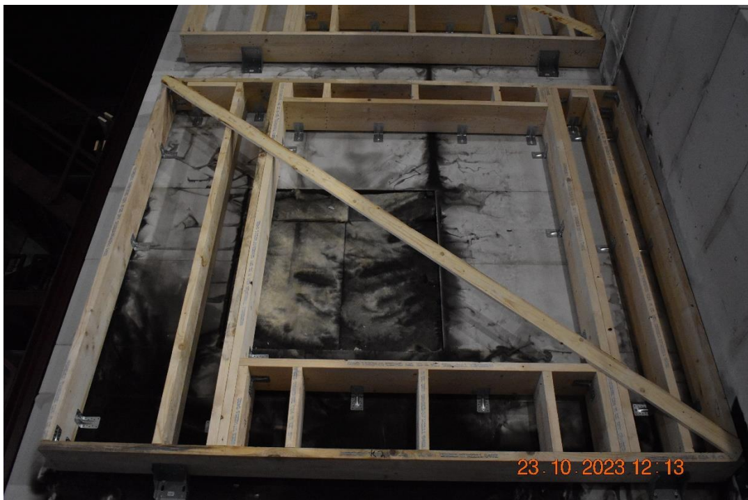
Photo No. 2 Fixing of prefabricated cassettes.
