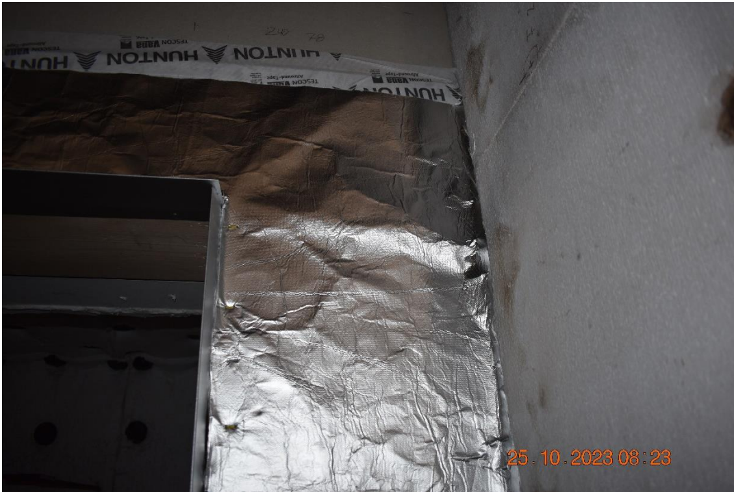
Photo No. 9 Traspir alu 430 mounted to the prefabricated cassettes.
