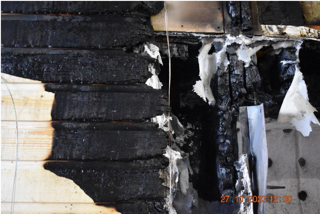
Photo No. 31 Test specimen after the test. Detailed photo of cladding and the cassette at the right side of fire chamber.
