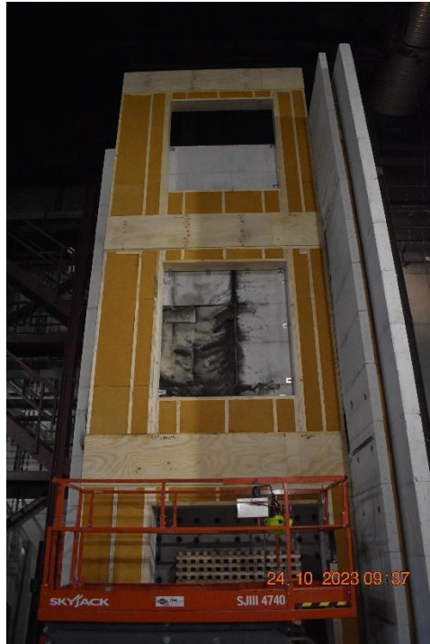
Photo No. 5 Isolation layer applied to the façade.
